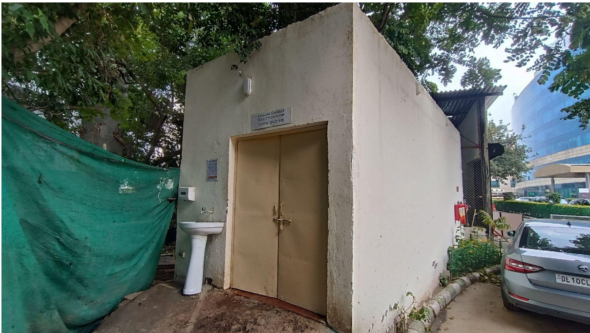
Photograph :- Solid-Waste Storage Room
