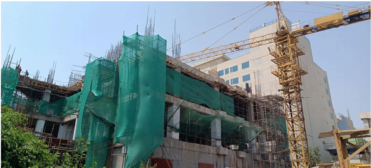
Photograph :- Under-Construction Building
